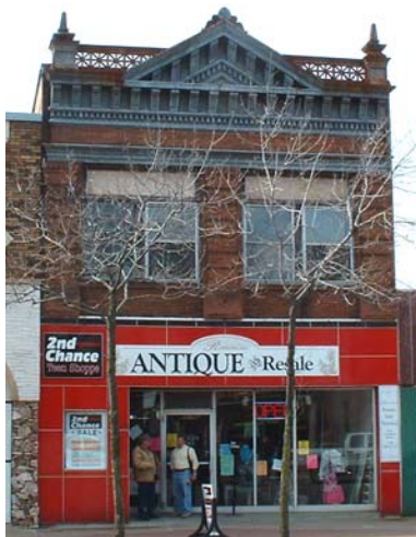
1215 Ludington before renovation
